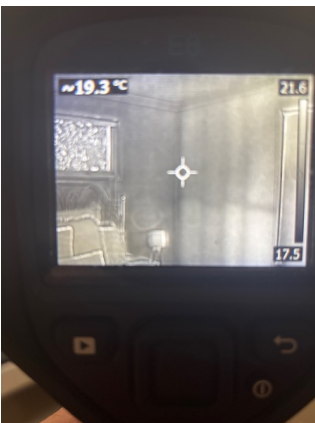
Thermal imaging of internal wall with no abnormalities
